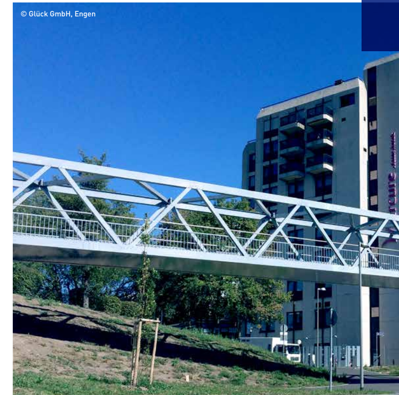
Figure 2: Aluminium bridge construction for the 'Kongresssteg Saarbrücken' project
